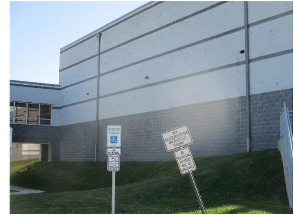
A rain garden can be installed in the turfgrass area on the west side of the building and on the turfgrass area in the parking lot to capture, treat, and infiltrate stormwater runoff from the roof. Parking spaces north of the building can be replaced with pervious pavement to capture and infiltrate stormwater runoff from the parking lot. A preliminary soil assessment suggests that more soil testing would be required before determining the soil's suitability for green infrastructure.
